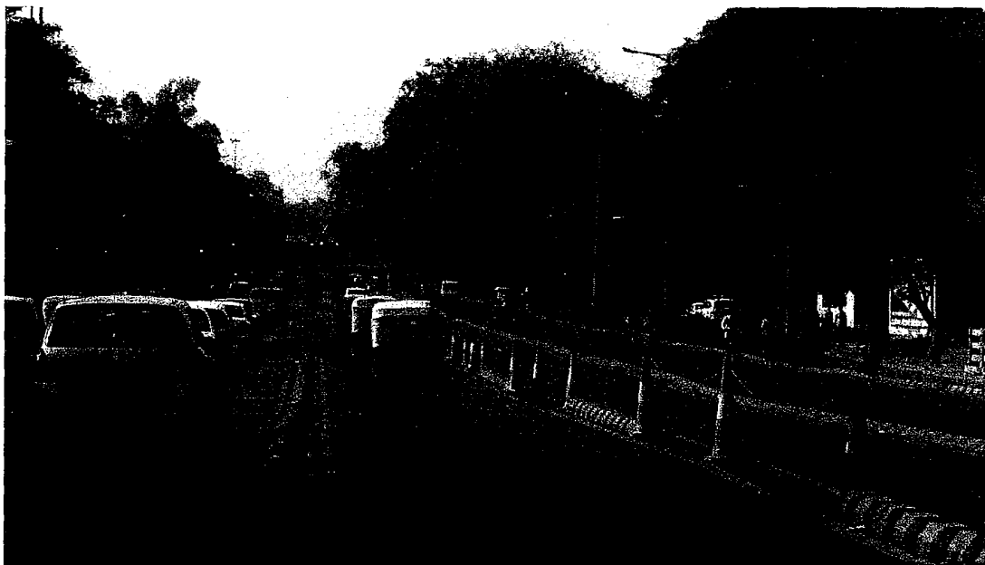
Photo 5.3.9: Temporary barricading to control the traffic in Opposite Lanes during the Experimental Trial Run
